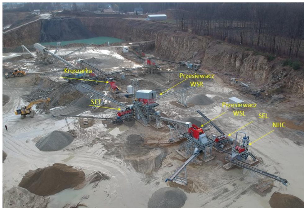
Rys. 2. Linia technologiczna w Kopalni Dolomitu Imielin, obraz z drona Fig. 2. Technological line in the Imielin Dolomite Mine, image from a drone
