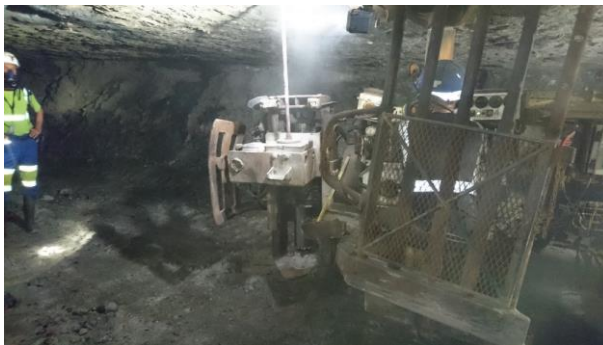
Bolting for supporting
