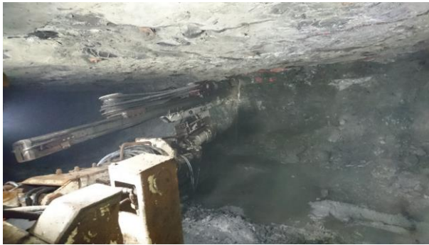
Drilling for blasting
