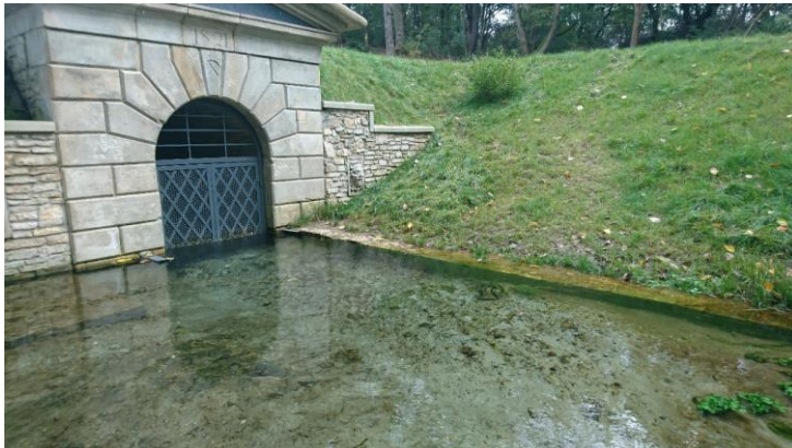
Part of the Historic silver mine drainage system
