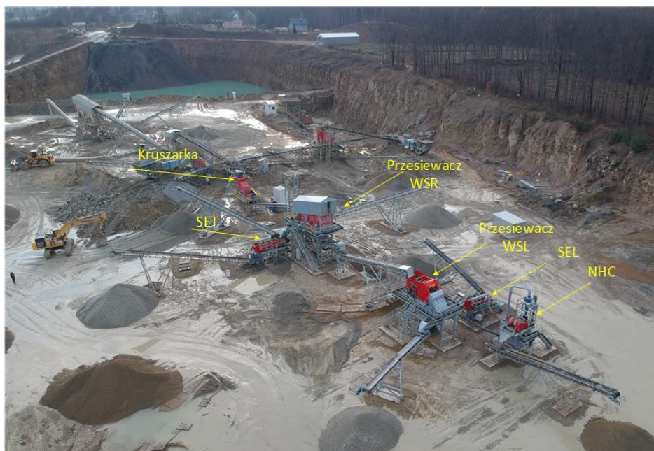
Rys. 3. Linia technologiczna w Kopalni Dolomitu Imielin, obraz z drona Fig. 3. Technological line in the Imielin Dolomite Mine, image from a drone
